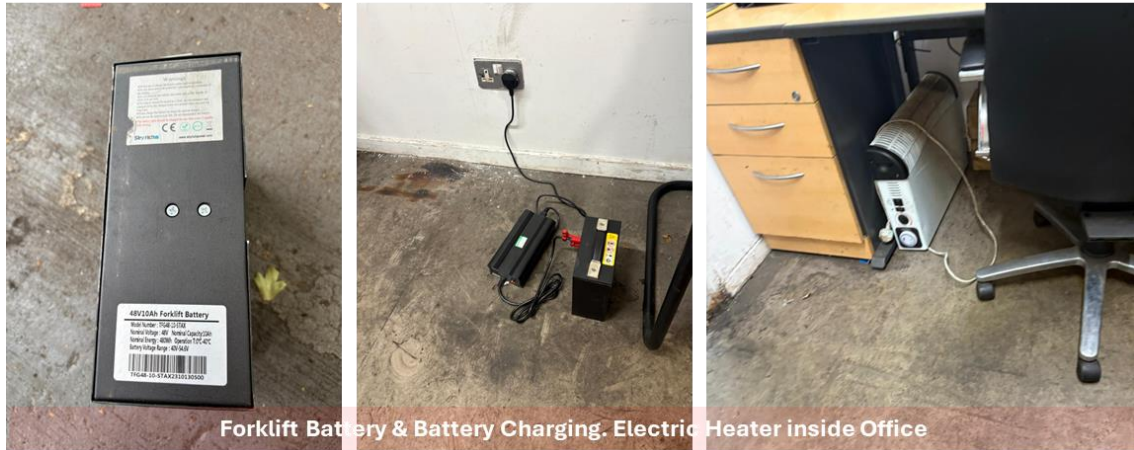
Figure 3 - Cleaning Station and Forklift Battery Charging
